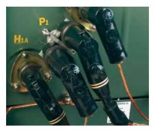
Two elbow arresters and a feed-through This approach uses elbow arresters only. (One of the elbow arresters may be mounted on the H1A bushing if operating procedures permit.)
