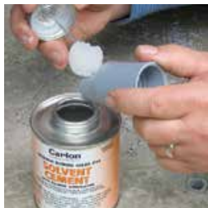
Apply a uniform coat of cement.
