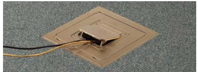
Flush mounting configuration. Optional trim ring allows cover to be mounted flush with tile or wood floors.
