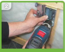
Screw the box to the stud using the center hole.
