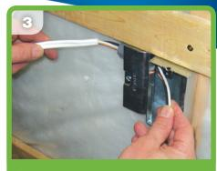
Insert the cable into the box.
